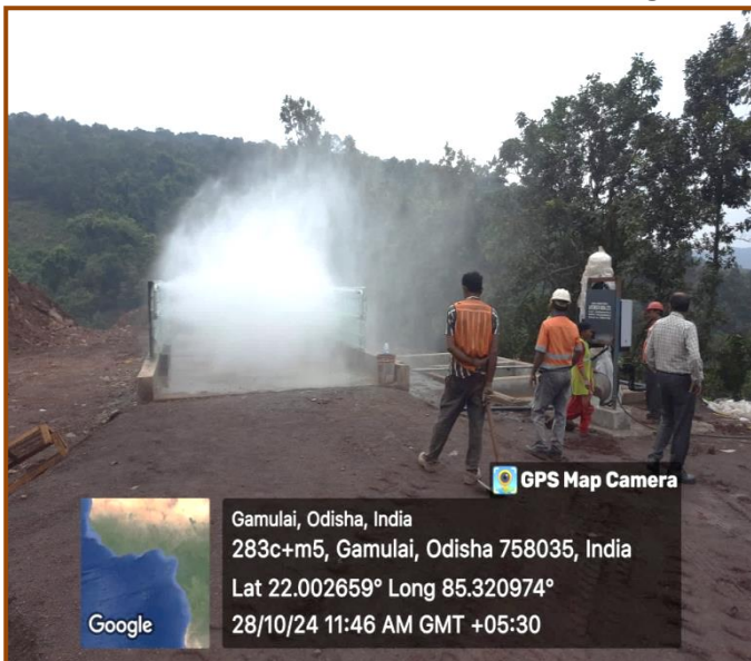
Photo-4 Wheel Wash Facility near exit gat
